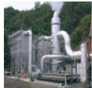
Incineration unit using a dioxin removal system
