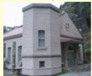
Ota Power Station
