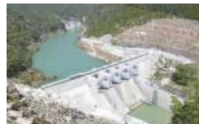
Test flooding of lower dam
