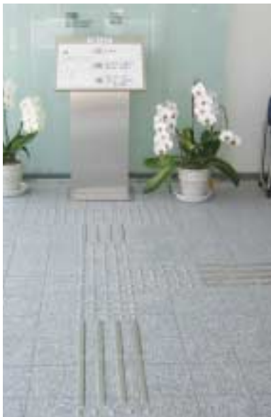
▼Textured pavement for guidance
