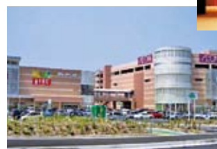
AEON Ito Shopping Center (Air conditioning ducts)
