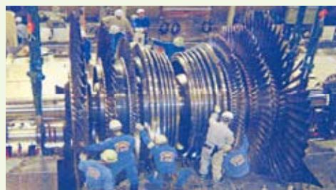
▲ Replacing a turbine at The Sendai Nuclear Station Unit 1
