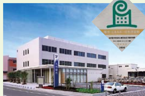
Exterior of Kirishima customer service office (opened on February 27, 2006)
