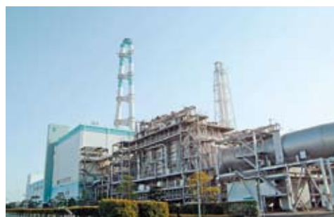
LNG-fired Shin Oita Power Station
