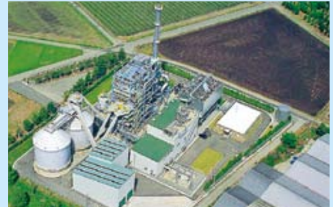
Miyazaki Biomass Recycle Co., Ltd. in Miyazaki Prefecture
