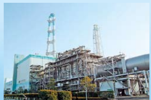
LNG-fired Shin Oita Power Station
