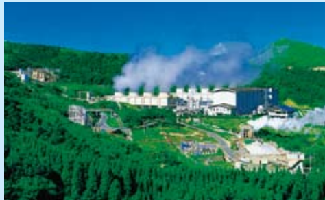
Hatchobaru Geothermal Power Station in Kokonouecho, Oita Prefecture
