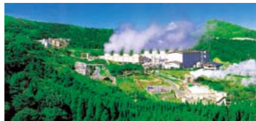
Hatchobaru Geothermal Power Station
