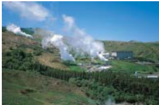
Hachchoubaru Geothermal Power Station
