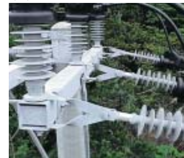
Polymer insulator for 22kV distribution lines
