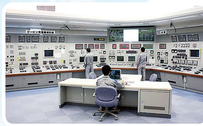
Simulator room in Genkai Nuclear Power Station training center
