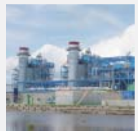
THE TUXPAN NO. 5 PROJECT
