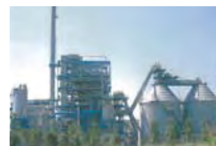
Miyazaki Poultry Manure Incineration Power Station (Miyazaki Biomass Recycling Co., Inc)
