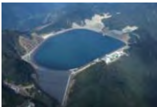
Omarugawa Power Station
