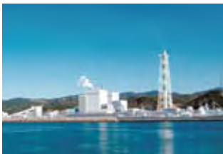
Reihoku Power Station
