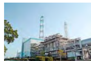
Shin Oita Power Station
