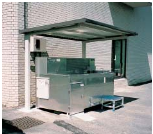
Composting facility installed at Education & Training Center
