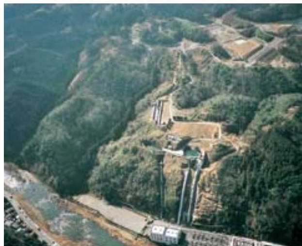
Bird's-eye view of Onagohata Power Station
