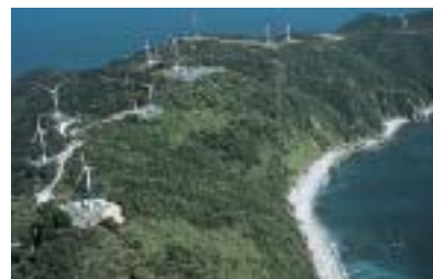
Cape Noma Wind Park Power Station
