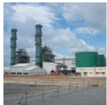
Phu My Unit 3 IPP, Vietnam (under construction)
