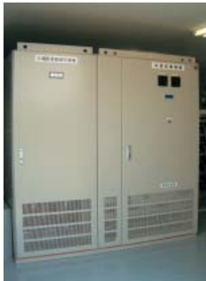
(Bidirectional converter and system interconnection protective board)
