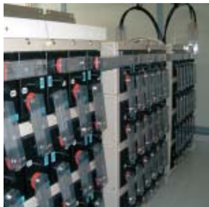
(LL lead storage battery)
