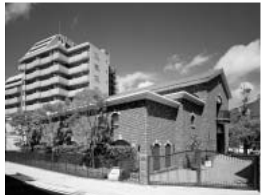
Shinchi Substation won a prize at the 12th competition of urban view plans of Nagasaki City
