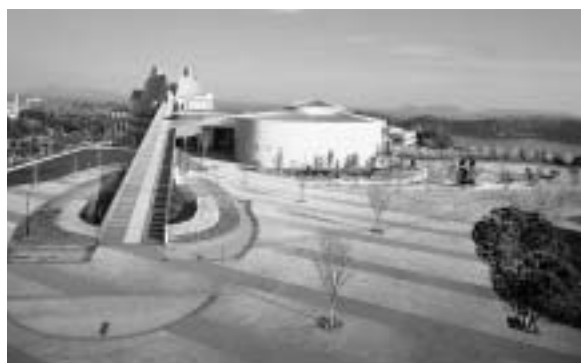
Genkai Energy Park (opened inside Genkai Nuclear Power Station premises March 31, 2000)
