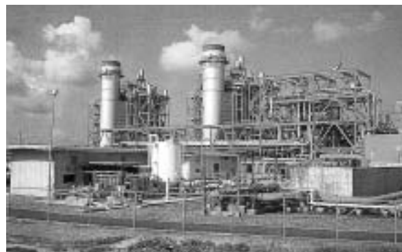
Tuxpan Unit 2 IPP, Mexico
