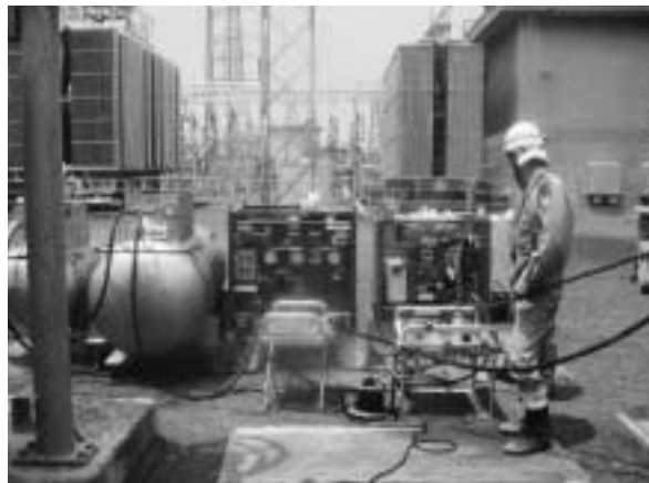
SF 6 gas recovery work
