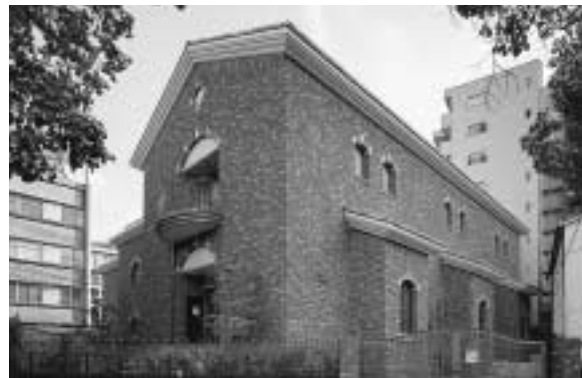
Shinchi Substation (Nagasaki City)
