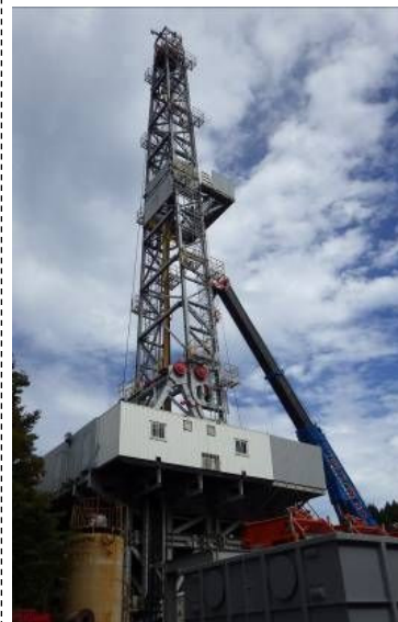
2,000m超を掘削
