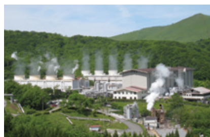
Hatchoubaru Geothermal Power Station
