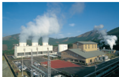
Takigami Geothermal Power Station
