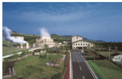
Ogiri Geothermal Power Station
