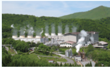
Japan's largest geothermal power station [Hatchobaru Geothermal Power Station]
