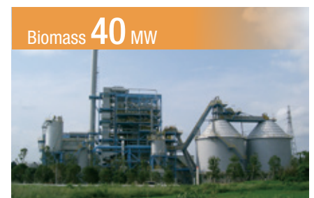
Biomass 40 MW Miyazaki Biomass Recycle Power Station Location: Miyazaki Prefecture Capacity: 11.35 MW Start of operations: May 2005
