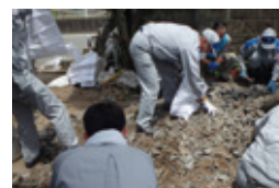
Removing broken roofing tiles
