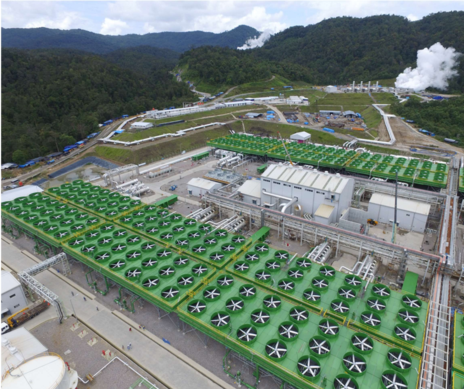
[The Second Unit of Sarulla Geothermal IPP Project in Indonesia]
