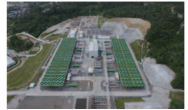
Aerial view of Sarulla Geothermal Power Plant Unit 1
