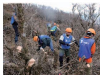
Clearing obstructing trees
