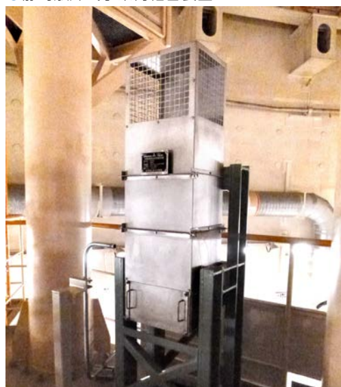
● 静的触媒式水素再結合装置
