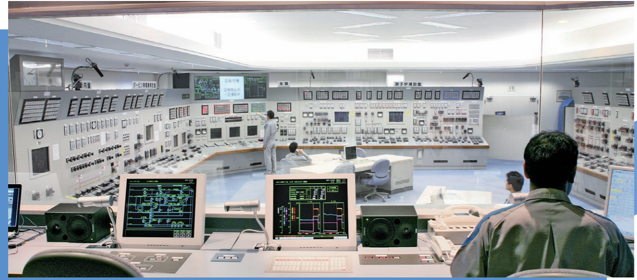
Instructor room (2-loop operation)
