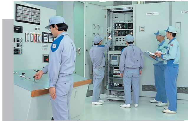
Control rod drive mechanism control system (Training in understanding the functions of the control rod drive mechanism control system, and in maintenance and inspection.)
