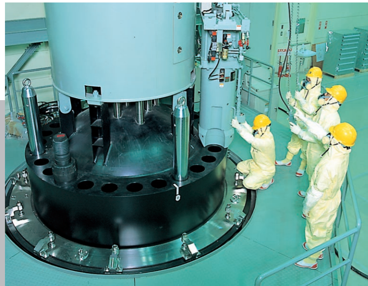
Reactor vessel head mock-up (Training in opening, inspecting and restoring the reactor vessel head.)
