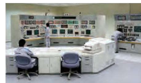
Simulator room (for units 3 and 4)
