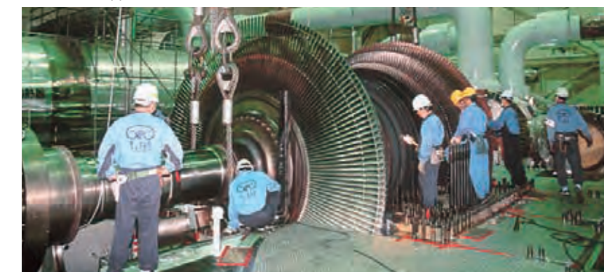
Overhaul inspection of turbine
