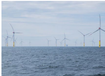
RWE Renewables' Arkona Offshore Wind Power Station (Germany)
