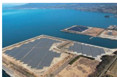
Omura Mega Solar Power Station
