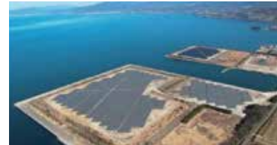
Omura Mega Solar Power Station
