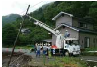
Introduction of restoration work after heavy rainfall in July 2020
