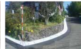
Support for improvement of access roads, etc. (placement of covers on gutters)
