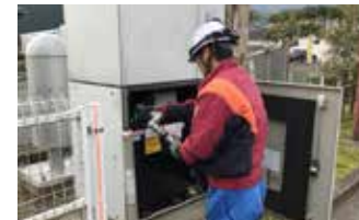
Fuel supply support for monitoring post
