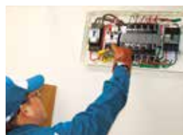
Inspection of distribution boards
