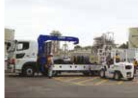
Transport of power cables
