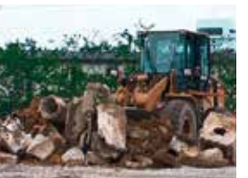
Removal of debris by heavy machinery
