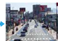
After the removal of utility poles
