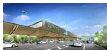
Kumamoto Airport new terminal building (to open in spring 2023)
