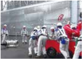
Placement of water cannon
