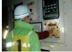
Power supply by high-voltage generator truck (nighttime)
