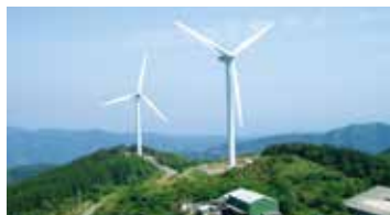
Nagashima Wind Power Station
