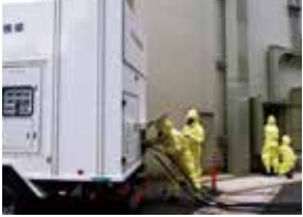
Connecting high-voltage generator truck power cables
