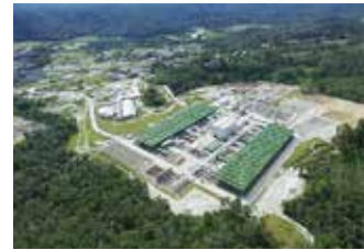
Sarulla Geothermal IPP Project
