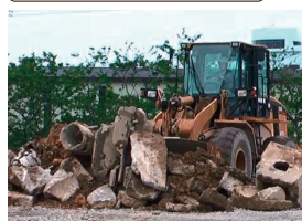
Removal of debris by heavy machinery
