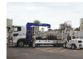
Transport of power cables
