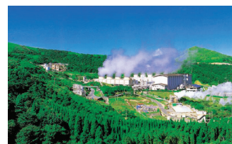
Hatchobaru Power Station
