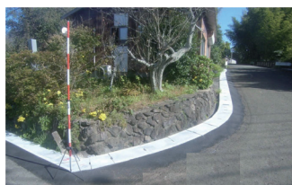
Support for improvement of access roads, etc. (placement of covers on gutters)
