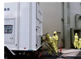
Connecting high-voltage generator truck power cables
