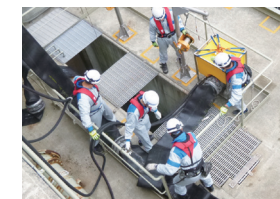
Installation of a submerged pump for drawing seawater
