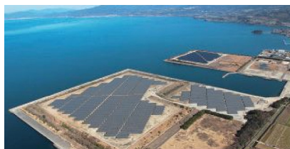
Omura Mega Solar Power Station
