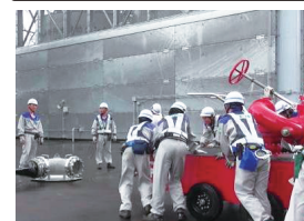
Placement of water cannon
