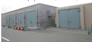
Storage facilities for materials and equipment (Genkai)
