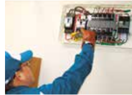
Inspection of distribution boards
