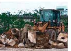
Removal of debris by heavy machinery
