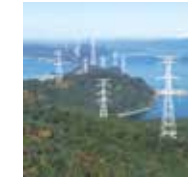
Power transmission towers
