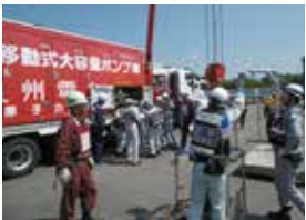
Placement of mobile large-capacity pump truck
