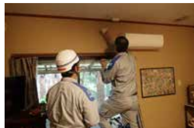
Indoor wiring diagnosis (Kumage Distribution Office)
