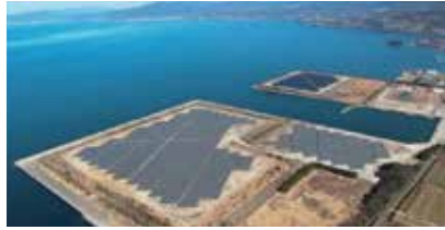
Omura Mega Solar Power Station
