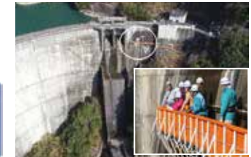
Visitors walking along the inspection walkway of Kamishiiba Dam, Miyazaki Prefecture
