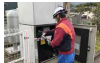
Fuel supply support for monitoring post
