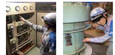
Checking instruments by pointing and calling | Checking for abnormal sounds with a stethoscope
