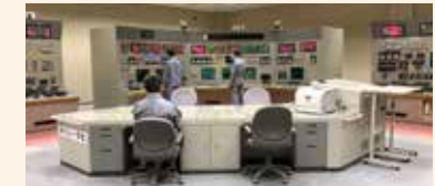
Simulator room at the Genkai Nuclear Power Station Training Center
