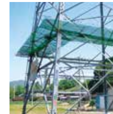
Installation of climbing prevention devices on power transmission towers
