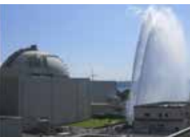
Water discharge by water cannon
