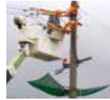
Use of fall prevention nets during work on power lines
