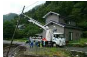
Introduction of restoration work after heavy rainfall in July 2020
