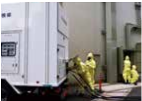
Connecting high-voltage generator truck power cables
