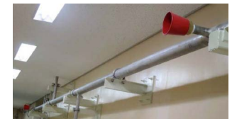
■ Automatic fire extinguishing system (Halon fire extinguishing system)
