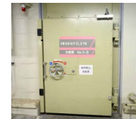
■ Overflow countermeasures (watertight door)
