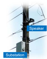
Installation on utility poles
