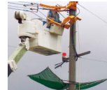
Use of nets to prevent falls during power distribution work
