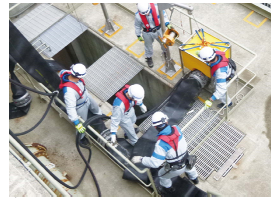
◇Installation of submersible pumps to intake seawater
