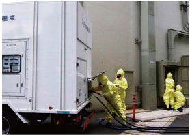
◇Connection high-voltage generator truck power cables
