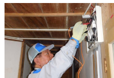
Indoor wiring inspection (Kumage Distribution Office)
