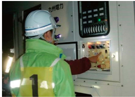
◇Power supply using a high-voltage generator truck (at night)
