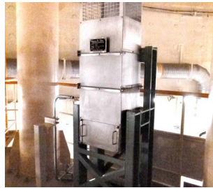
■ Static catalytic hydrogen recombination device
