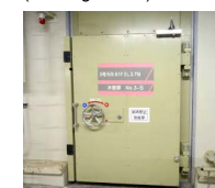
Overflow countermeasures (watertight door)
