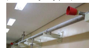
Automatic fire extinguishing system (Halon fire extinguishing system)
