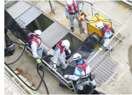
Installation of submersible pumps to intake seawater
