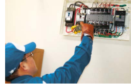
Distribution board inspection
