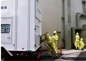
Connection high-voltage generator truck power cables
