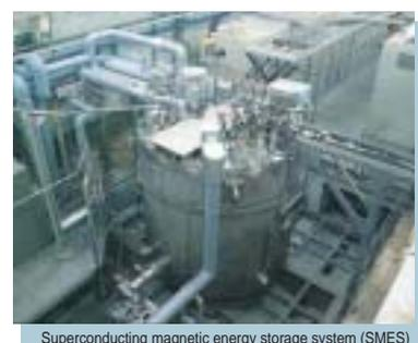
Superconducting magnetic energy storage system (SMES)
