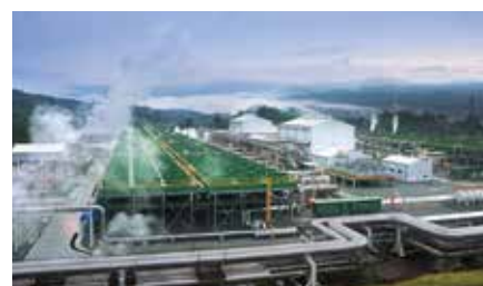
Unit 1: Operation commenced March 2017 Unit 2: Operation commenced October 2017 Unit 3: Operation commenced May 2018
