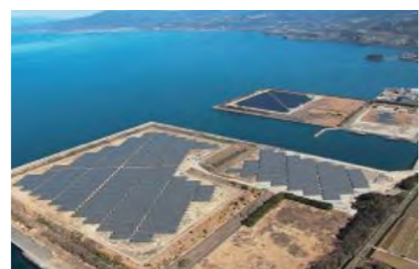
Omura Mega Solar Power Station
