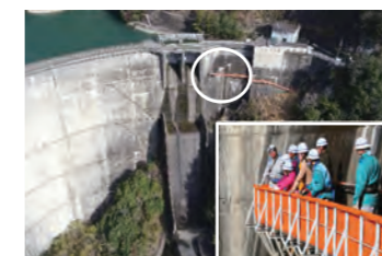
Walking tour of inspection passageways at Kamishiiba Dam, Miyazaki Prefecture
