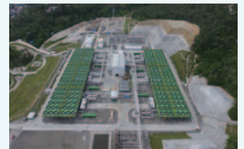
Aerial view of Sarulla Geothermal Power Plant Unit 1
