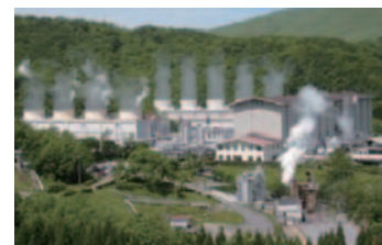
Hatchobaru Power Plant
