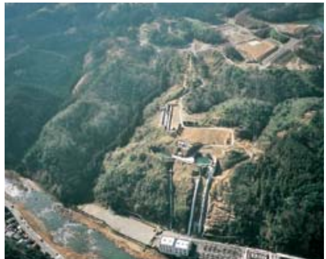
Bird's-eye view of Onagohata Power Station
