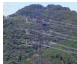
Steel tower painted to be in harmony with the environment
