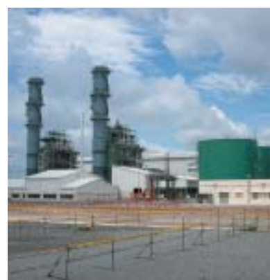
Phu My Unit 3 IPP, Vietnam (under construction)
