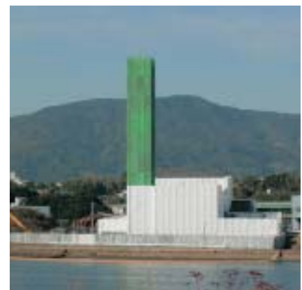
(Dismantling works of the former Tobu Clean Center in Sasebo City)
