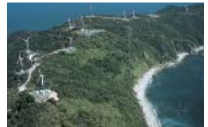
Cape Noma Wind Park Power Station
