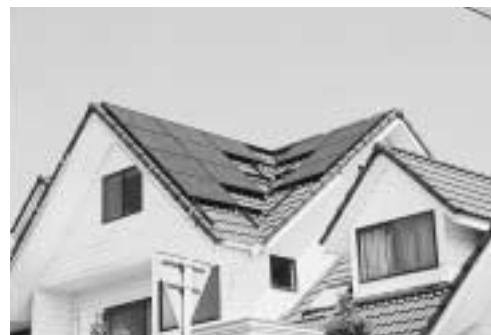
Installation of photovoltaic power generation panels
