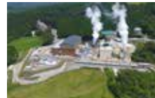
Otake Power Station
