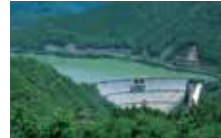
Hitotsuse Power Station
