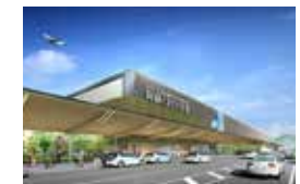
Kumamoto Airport New Terminal Building (to be operational in spring 2023)
