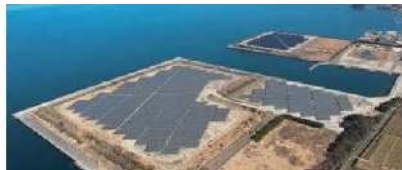
Omura Mega Solar Power Station (Kyuden Mirai Energy)
