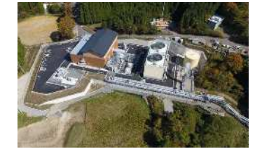
Geothermal power business: Otake Power Station
