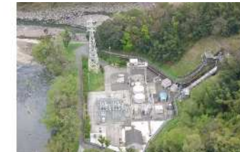
Hydro power business: Shintakeda Power Station
